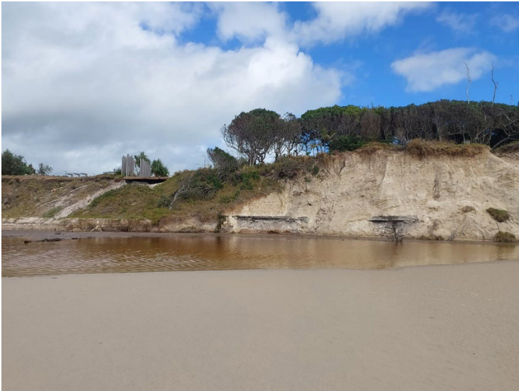
Photo1: Site of proposed coastal protection works is the eroded (and grassed) face to the left of the photo. The eroded dune to the right (northwest of the proposed works) has an unstable face approximately 5 metres high, revealing a Pleistocene soil profile at the base of the dune, overlain by cross-bedded sand deposits with no soil profile development. Belongil creek currently flows across the base of this eroded dune face, which continues to slump.
